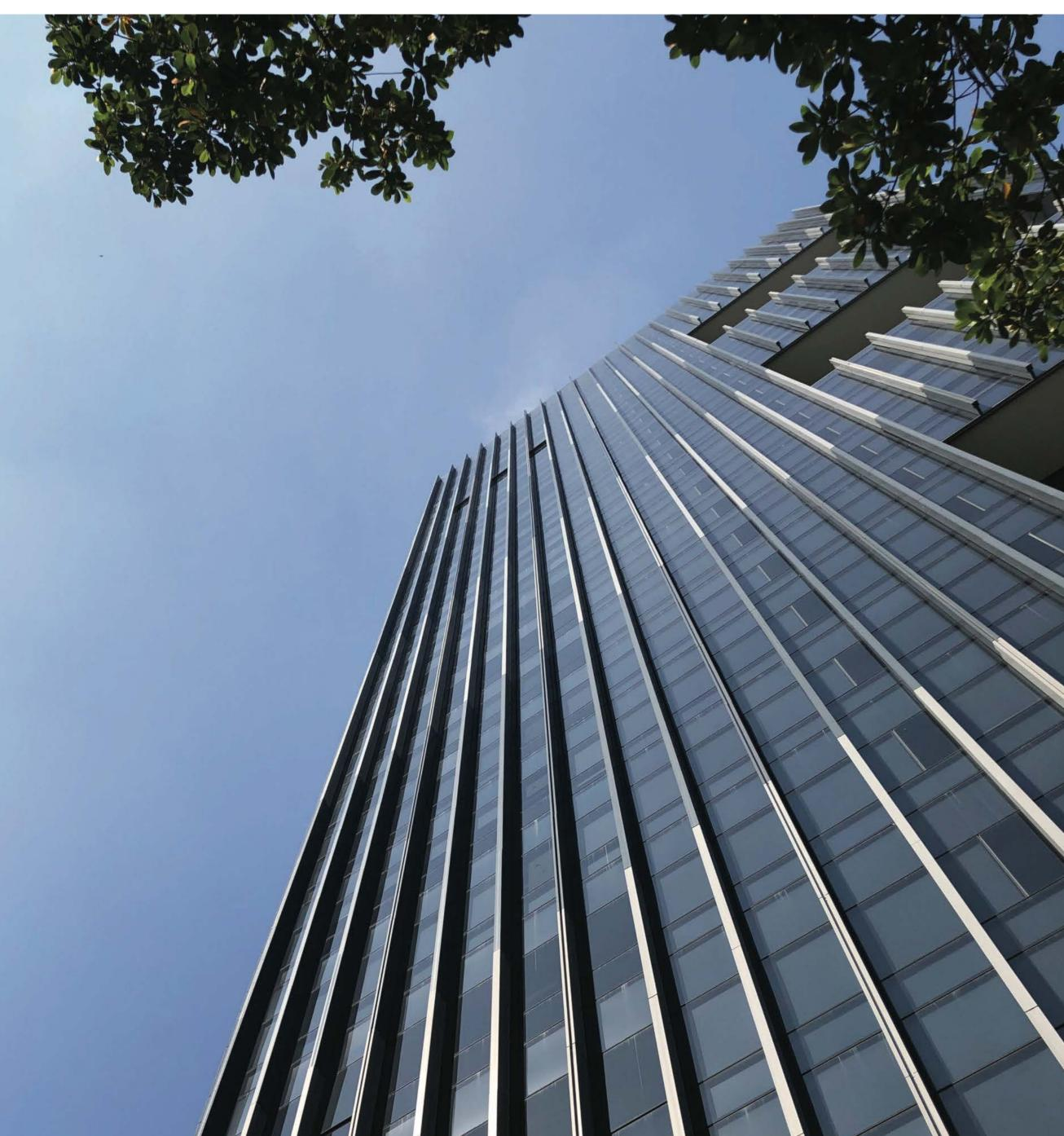
**Nucleus Tower** "We designed Nucleus Tower, a high-end corporate office building in Mutiara Damansara, with a green building approach that responds to the environment," says Harzani. "The building facade is completed with shading devices for all curtain wall openings. In addition to featuring multi- and single-tenant office spaces in the
